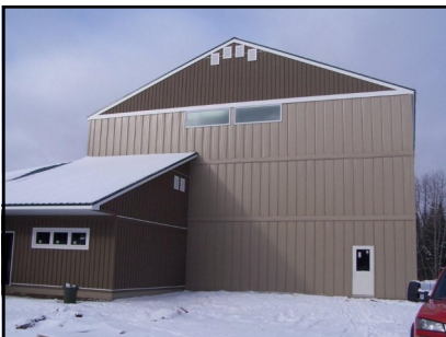
Phase 1 of the Keekanaw Multi-purpose Facility has been completed.
